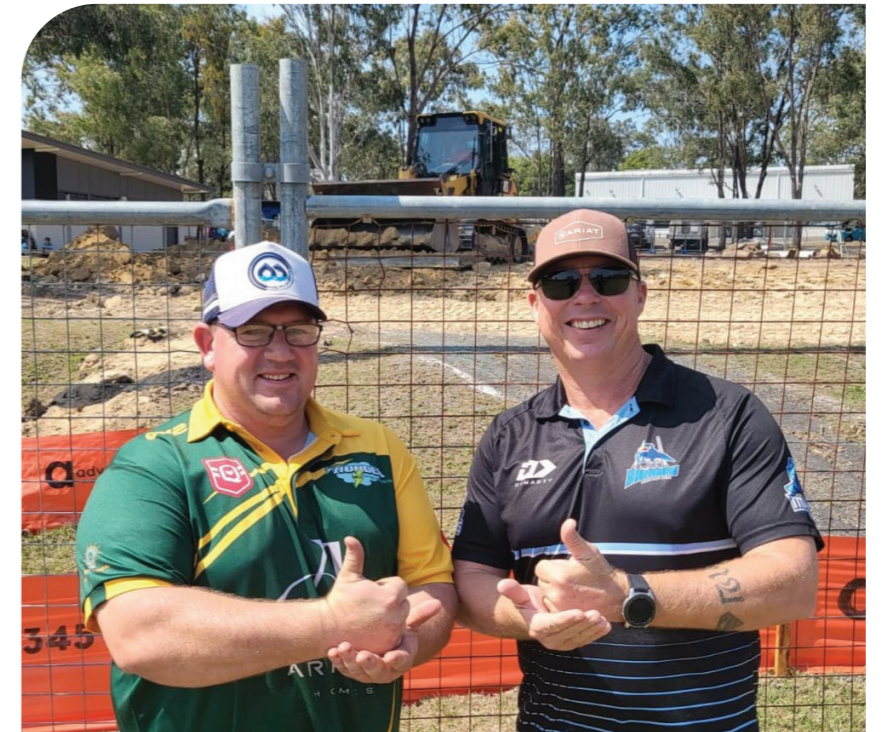
Cr Scott Bannan with Matt from Jimboomba Junior Rugby League Club, celebrating the start of construction on the new clubhouse.
