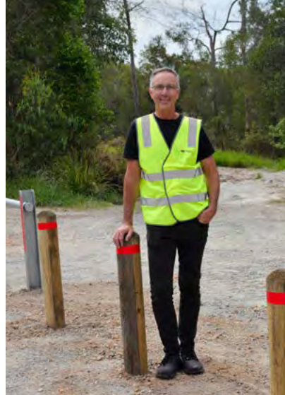
Cr Paul Jackson inspects the new bollards installed to combat illegal dumping in Berrinba.
