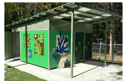
The new amenities block in Forestglen Park at Browns Plains.
