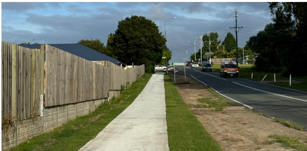
Construction of the new Heritage Park footpath, now completed.
