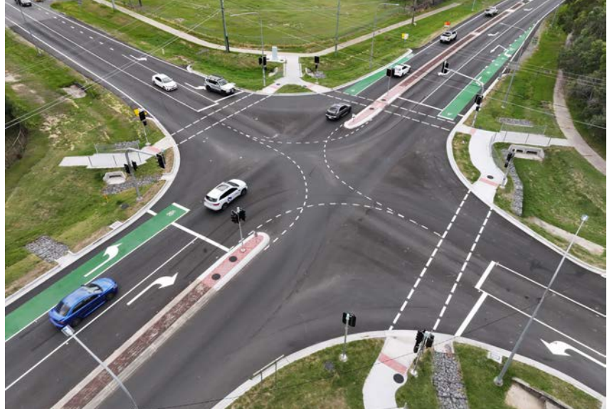
Traffic flow is improved now Council works are complete at the new Park Ridge intersection,
