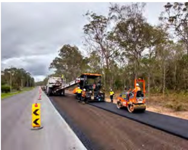
Work on the current stage of the Chambers Flat Road upgrade.
