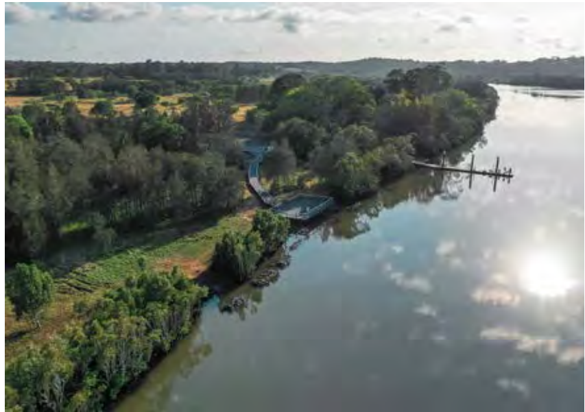
Aerial view of the new boardwalk and platform.
