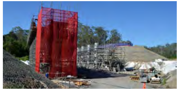
The Norris Creek bridge under construction.
