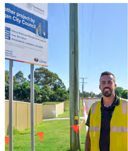
Cr Nathan St Ledger outside Logan Village State School during the construction works.
